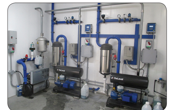
Figure 1. Equipment room free of clutter, dust and debris.
