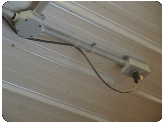
Figure 2. Temporary electrical equipment plugged into receptacle in livestock area.
