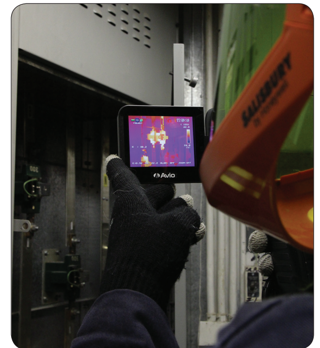
Figure 5. Inspection of electrical equipment by insurance company.
