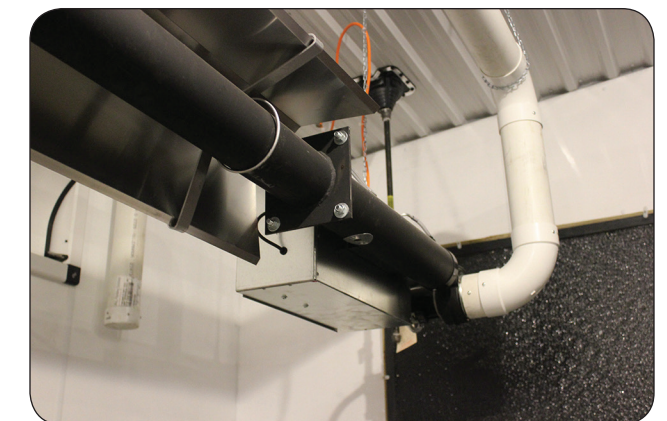
Figure 8. Radiant tube heater suspended in barn.
