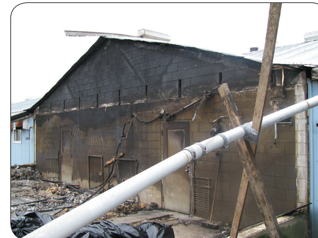
Figure 7. Example of an intact fire separation that did its job and prevented fire from spreading through the barn.
